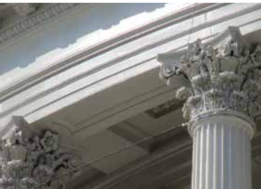
StealthNet prevents birds from roosting on the decorative columns of this historic building.
