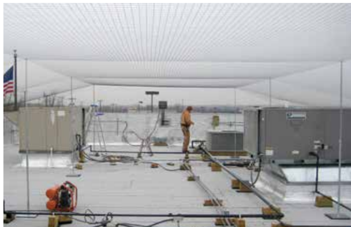
The telescopic support poles allow netting to be installed securely over the heads of workers and equipment.
